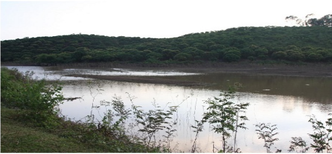
Figure 5 Inability to store design water capacity because of leakage
